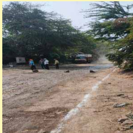
Levelling work & Metal laying Initiated..by MIDC
