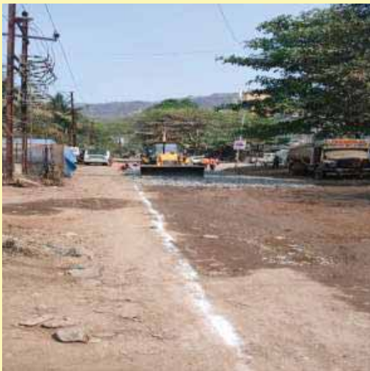
Levelling work & Metal laying Initiated..by MIDC
